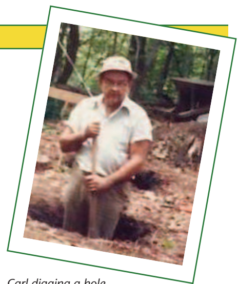
Carl digging a hole for an Appalachian Trail shelter pier.
