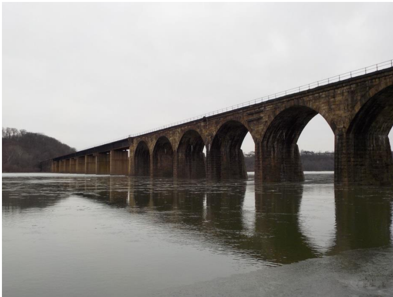
Shock's Mill Bridge from Lancaster Side
